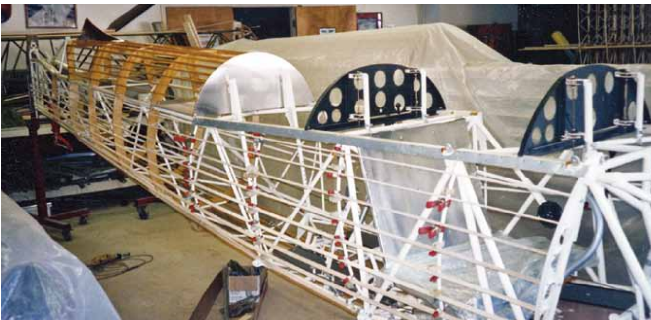
New wood stringers and formers on the fuselage in March 2003.
